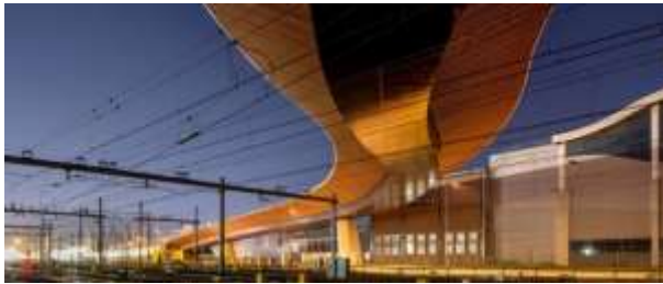
Figure 4: ESDA 2021 Special Bridge Award: Schuttebusbrug, Zwolle Photo: ipv Delft / Henk Snaterse
