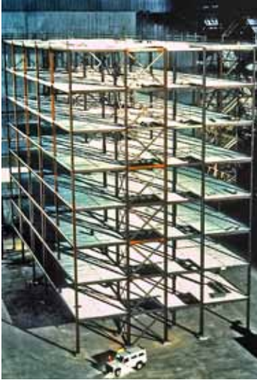
3.27 Cardington test building prior to concreting of the floors, and indication of test locations.
