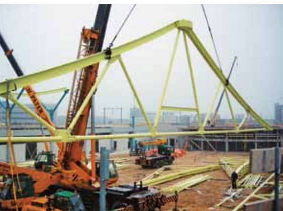
1.1 Use of large parts on the construction site.
