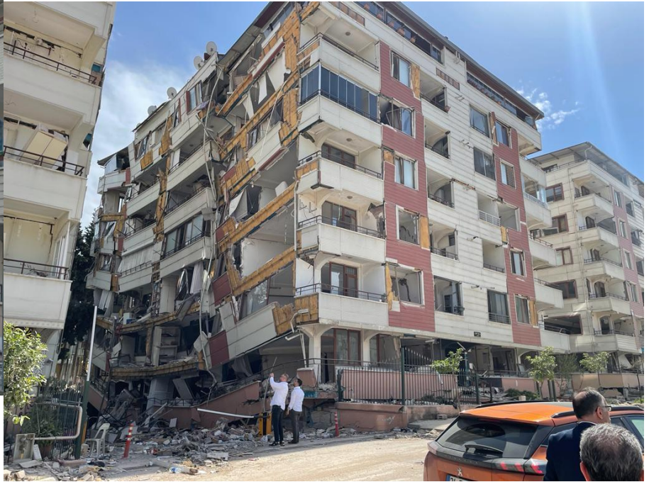
After the earthquake on 20 February
