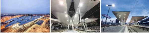
Central Railway Station - Diamond Shaped Roof, Vienna
