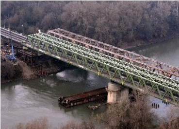
Renewal of Szolnok Railway Bridge, Szolnok
