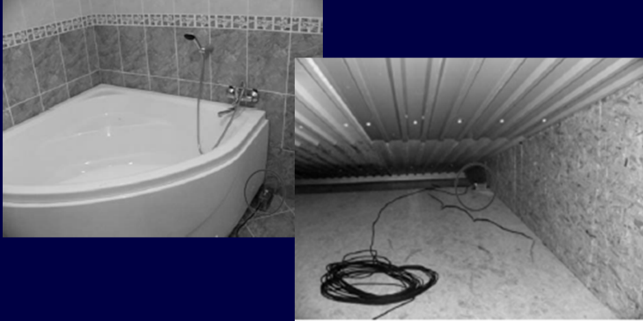
Construction Stage 3 and measurement sensor location
