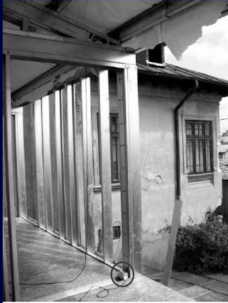
Construction Stage 1 and measurement sensor location on the skeleton of the structure
