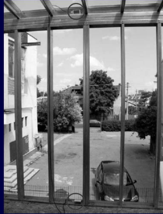
Construction Stage 1 and measurement sensor location on the skeleton of the structure
